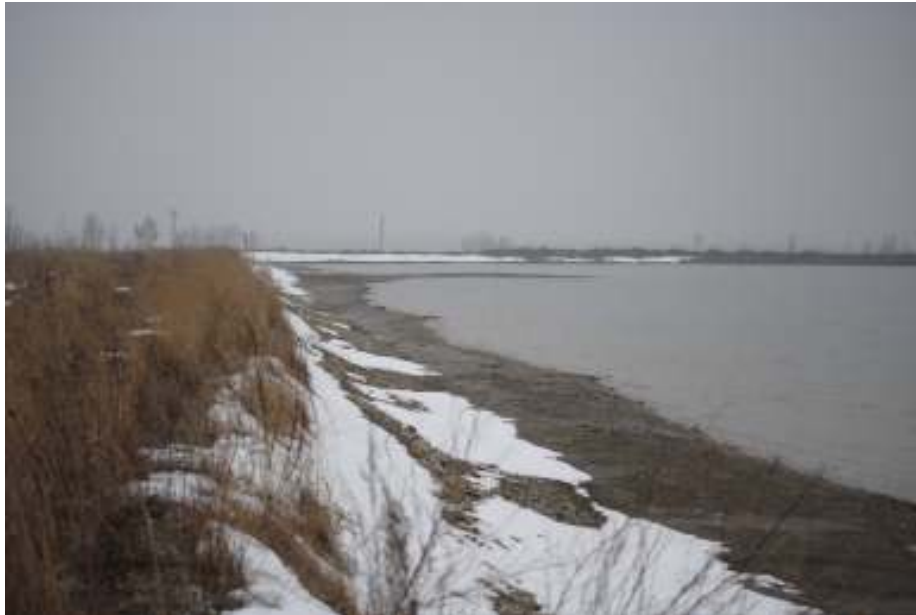
Figure 5: North side of Tailings Dam No. 2
