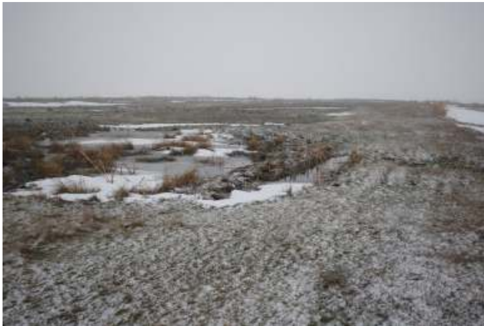
Figure 3: Grass cover on Tailings Dam No. 1
