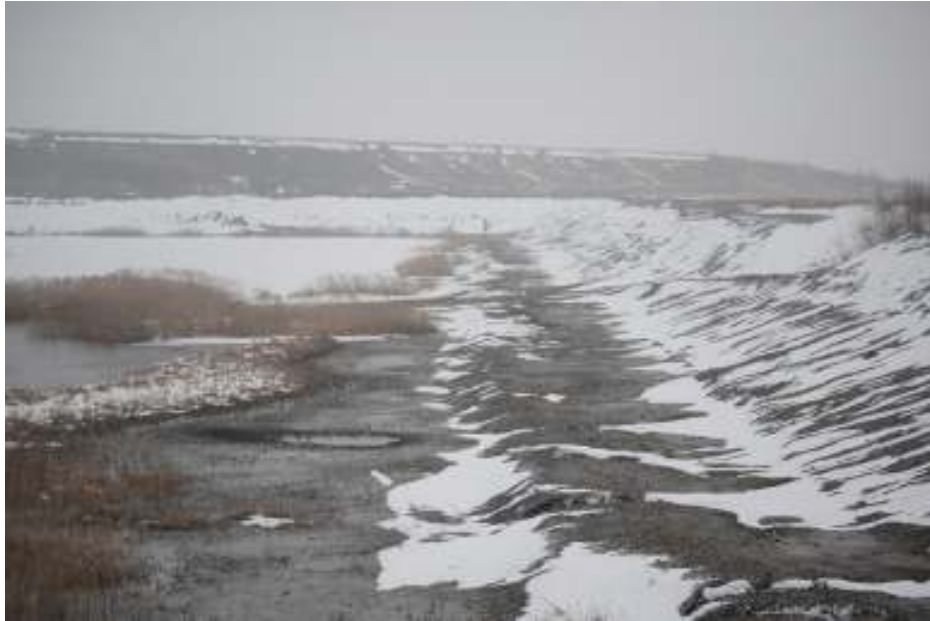
Figure 6: Start dam for Tailings Dam No. 3 (west side)
