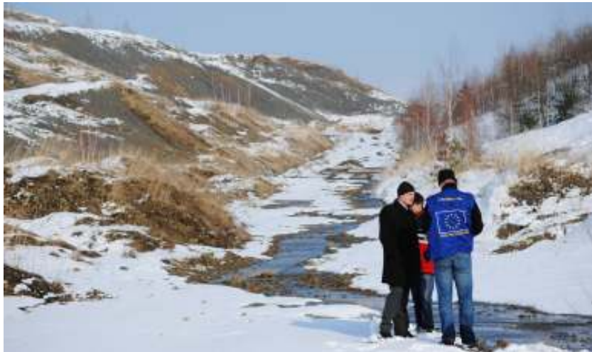
Figure 13: Surface discharge or brines on the east side of Waste Dump No. 1
