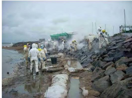
Example of high pressure washing with oily water recovery downstream in pits with sorbent, Loire estuary (France) 2008
