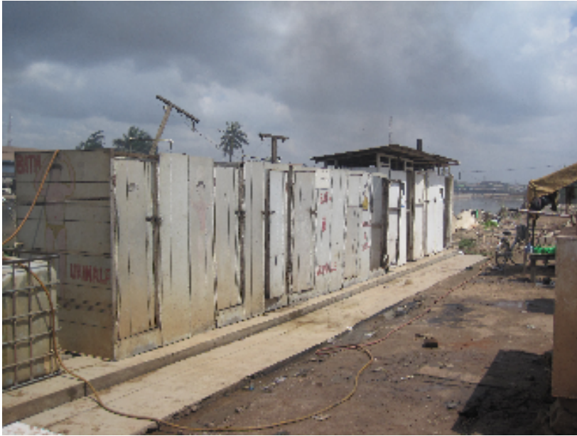
Public showers, urinals and toilets directly discharging into Odaw channel. Photo MSB
